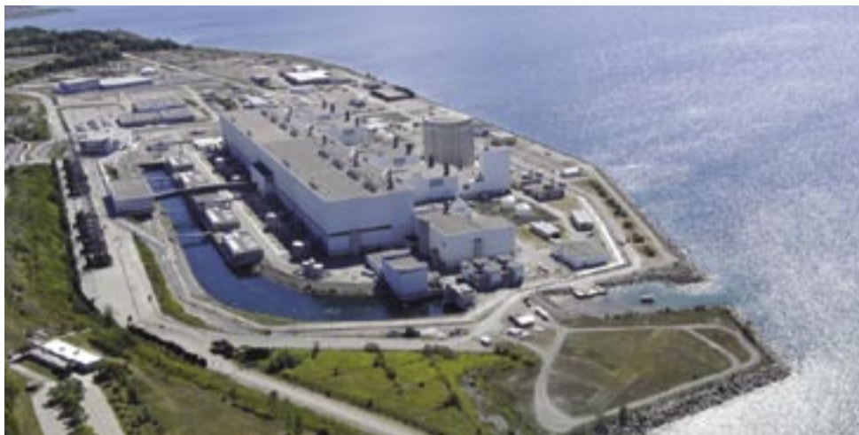
Ontario Power Generation's Darlington site will see the development of new reactors on its grounds.
